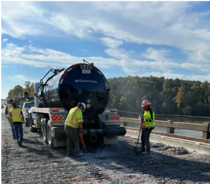
Figure 2: Rehab Work on US 321 Southbound Bridge over the Catawba River
