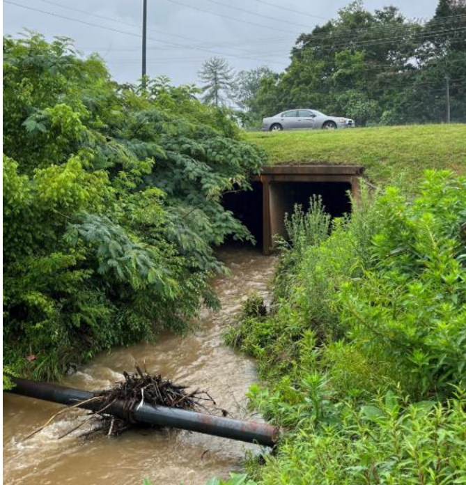
Figure 4: Frye Creek During a Rain Event
